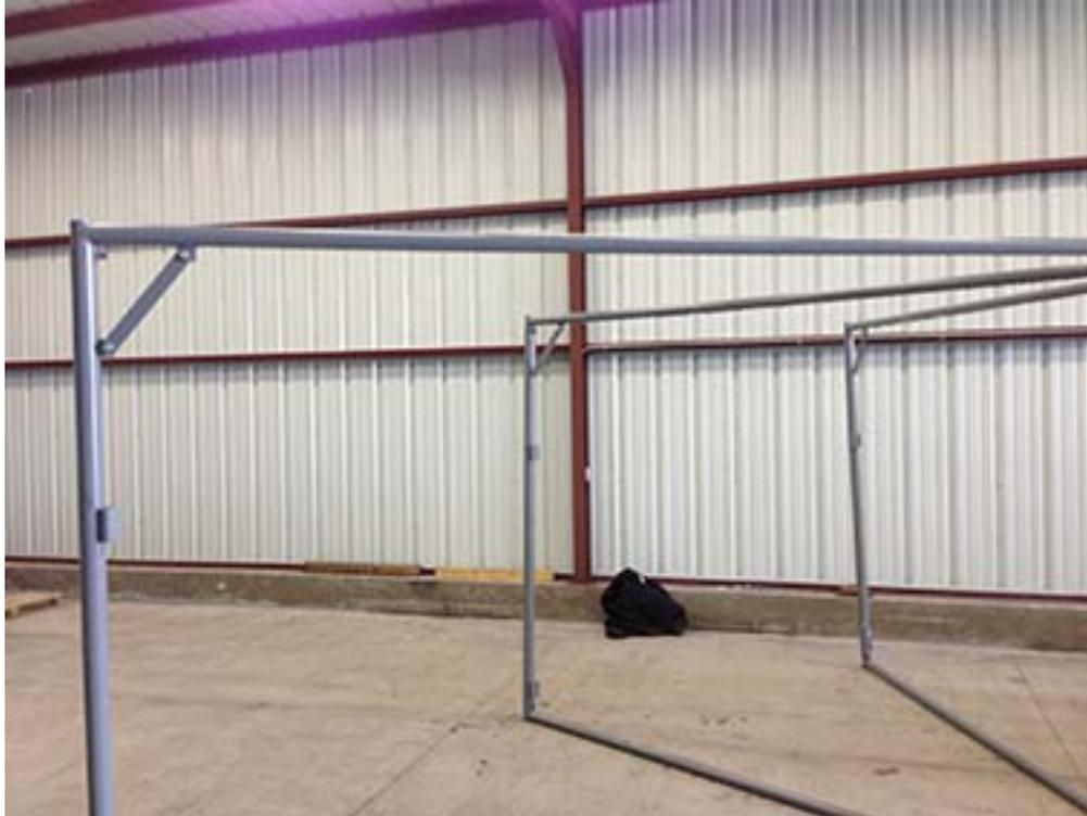
14. Pin the straight panel between the pivot pipe and the A frame by dropping four of the pins provided into the one inch pipes on the pivot pipe. Make sure smooth side is facing the inside of the tub toward the animals.
