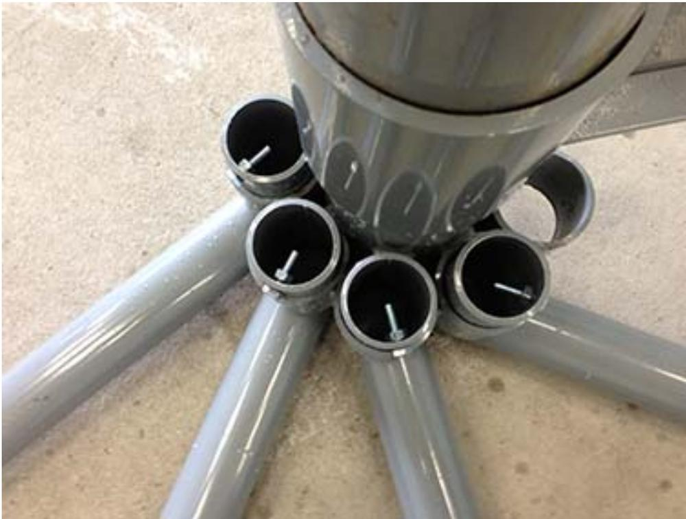
10. Place the A frame in position by placing the bottom collar over the stub pipe at the end of the remaining radial pipe.
